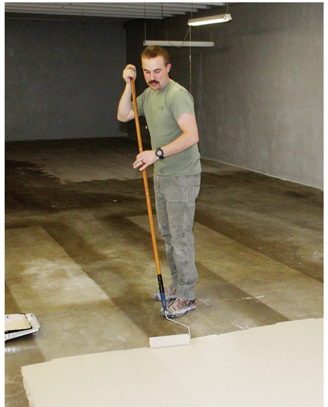
Photo by Walter Sprague/NLJ Zach Pickle paints the newly cleaned and prepared surface of the floor with added paint chips, giving the paint a better look and decreasing the slickness of the surface.
