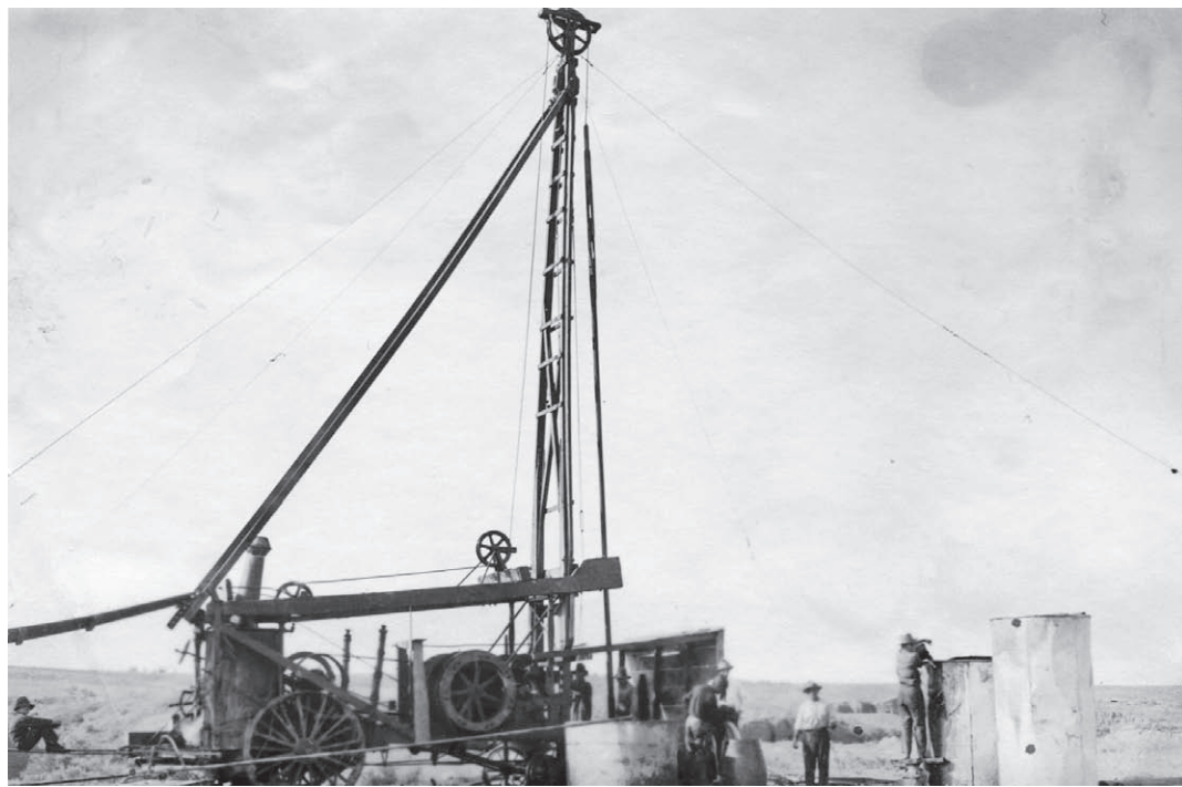
In March of 1920, a gusher oil well was struck in the Osage Oil Field. With the opening of the oil field people flooded to the area. By 1923, the oil boom went bust. In this 1920 photo, Muscrat Oil Company is drilling for oil in the Osage Oil Field, Sec. 17.
